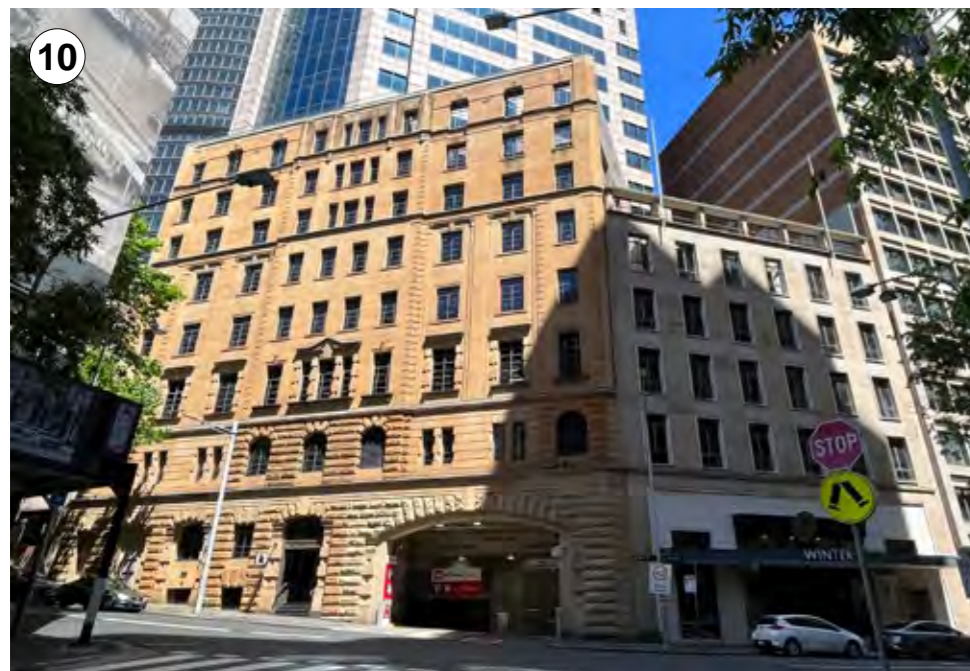
View of heritage facades to Bent and Spring Streets, with existing vehicle entry to basement within the larger Chatsworth House facade. The Orient Building facade visible in the lighter sandstone and to a lower height to the right.
