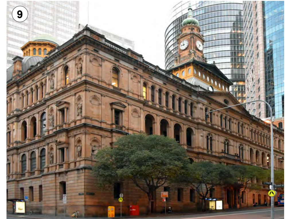
View of the western facing elevation of the Department of Lands Building. 1 O'Connell Street visible to the right, and the curved facade of 1 Bligh Street behind. The distinct copper onion-shaped clock tower forms a distinct landmark within the city (designed by colonial architect James Barnett). (Building currently covered in scaffold - image source: shorturl.at/jAKY0 .)
