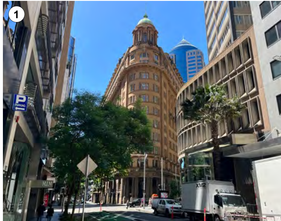
The Radisson Hotel (former Wales House) to the corner of Pitt Street and O'Connell Street and Hunter Street as viewed here from Pitt Street facing north. The iconic corner facade with copper dome is a distinct and well known city corner.
