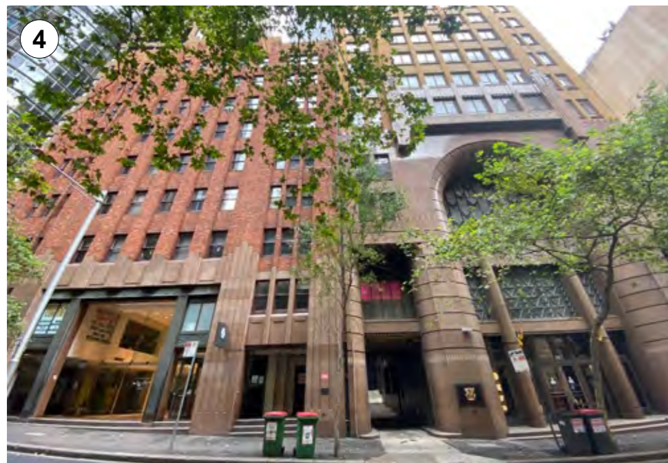
Opposite the site on O'Connell Street is 12-14 O'Connell Street former Manufacturer's House (left) and 16 O'Connell Street, Former Bank of NSW (right). 12-14 O'Connell has distinct Art Deco details with a sandstone base and red brick upper. 16 O'Connell Street has a granite base with sandstone upper and distinct decorative windows from ground to level 2.
