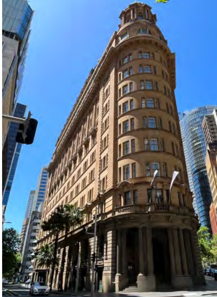
FORMER SYDNEY MORNING HERALD BUILDING AKA WALES HOUSE 66 Pitt Street (corner O'Connell Street) Completed: 1927 Architect: Manson & Pickering
