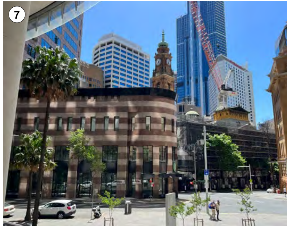
View of existing wintergarden building facing north-west, with the Department of Lands Building behind, taken from the steps of 1 Bligh Street (Department of Lands Building currently with scaffold covering the exterior). The existing post-modern wintergarden building design forms an acute point at the northern tip of the site.
